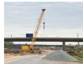
ROAD AND HIGHWAY CONSTRUCTION
