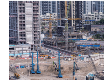
HIGH-RISE BUILDING CONSTRUCTION
