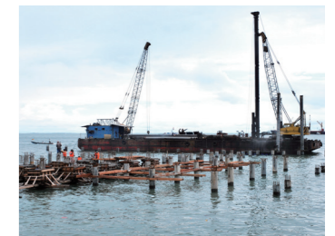
PORT AND DOCK CONSTRUCTION
