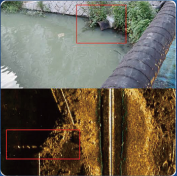
Subsurface Pipeline Inspection
