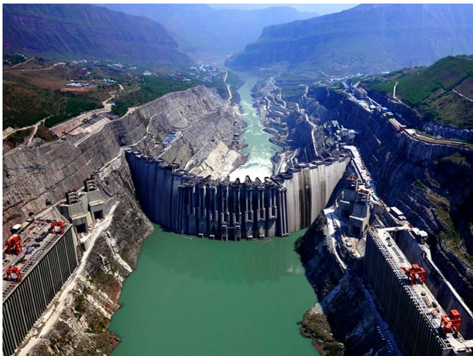
Xiluodu Hydropower Station
